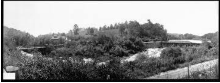
Hominy Creek Dam, 1915
